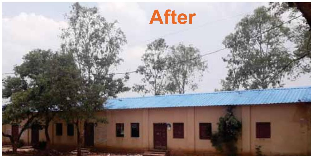
1) 10 Toilets, 2) 8 Class rooms - Replacement of asbestos sheets with tin sheets, new doors& windows, 3)132 steel taps and 4) 40 Fans.
