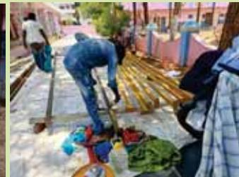
Next we have placed the girders and 'I' sections on pillars which we have layed from ground and those are being painted now and later we will place the sheds on the girders after painting work gets done sheds will be installed on the trusses, photos will be attached below
